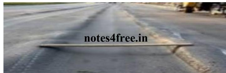
Fig.6: Real-Time Formation of Ruts
